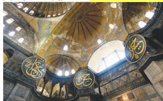
Recent innovation: triangular 'pendentives' join supporting arches to the building's enormous dome.
